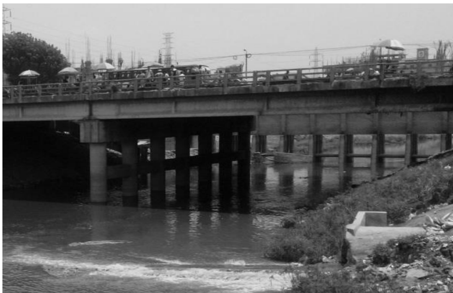
Figure 2: Rampura Regulator Gate Open
