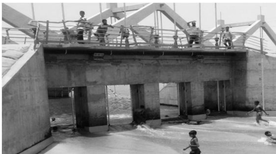
Figure 1: Hatirjheel Regulator Gate Open (Crest at an elevation of +2.5 m)
